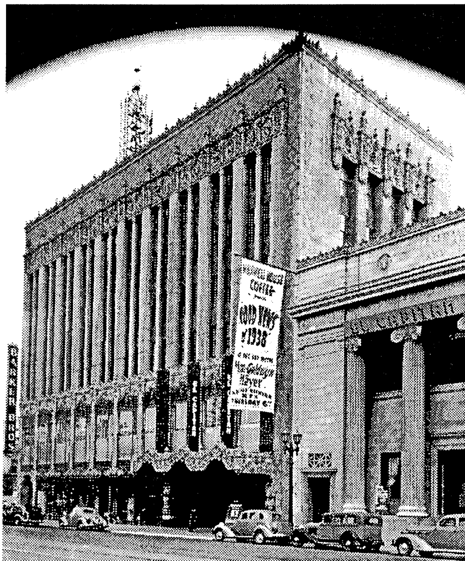
Figure 7-5 Existing buildings often incorporate a myriad of small gestures which catch and delight the eye. The El Capitan Theater at 6834 Hollywood Boulevard possesses decorative metal mullions which delineate projecting window bays, as well as ornamental metal and cast concrete elements.
