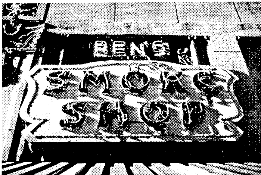
Figure 7-32 Historically, signs such as this example at 6423 Hollywood Boulevard and awnings were positioned within the building's structural bays.
